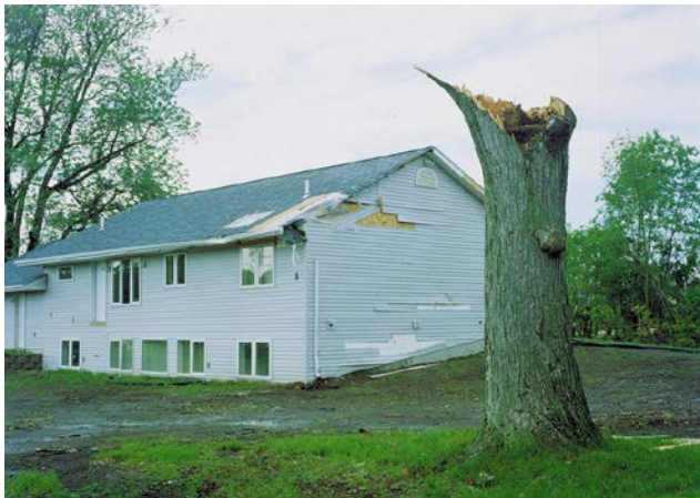
Figure 1: Tree impact to an ICF house with no damage to the ICF wall caused by the tornado.
